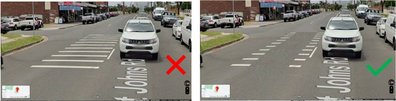
Figure 2. Example of incorrectly and correctly applied line marking in an urban street environment. In the image on the left, the lines have been installed to function as rumble strips, warning drivers of a hazard ahead. However, a driver exiting the side street may see stop lines and turn across or into the path of vehicles coming from the right, legitimately believing the vehicles on the right will stop. (Image on the right has been modified to demonstrate recommended altered line marking.)
