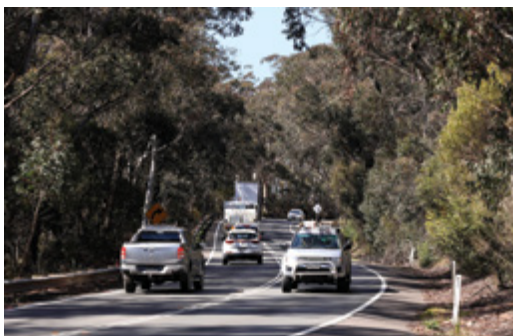
The project team are examining short term safety fixes that can be used at identified locations like Foy Avenue
