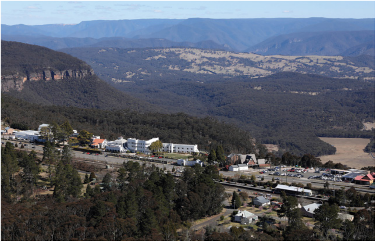
The proposed upgrade in Medlow Bath can be carried out within the existing road corridor with minimal impacts to property and environment
