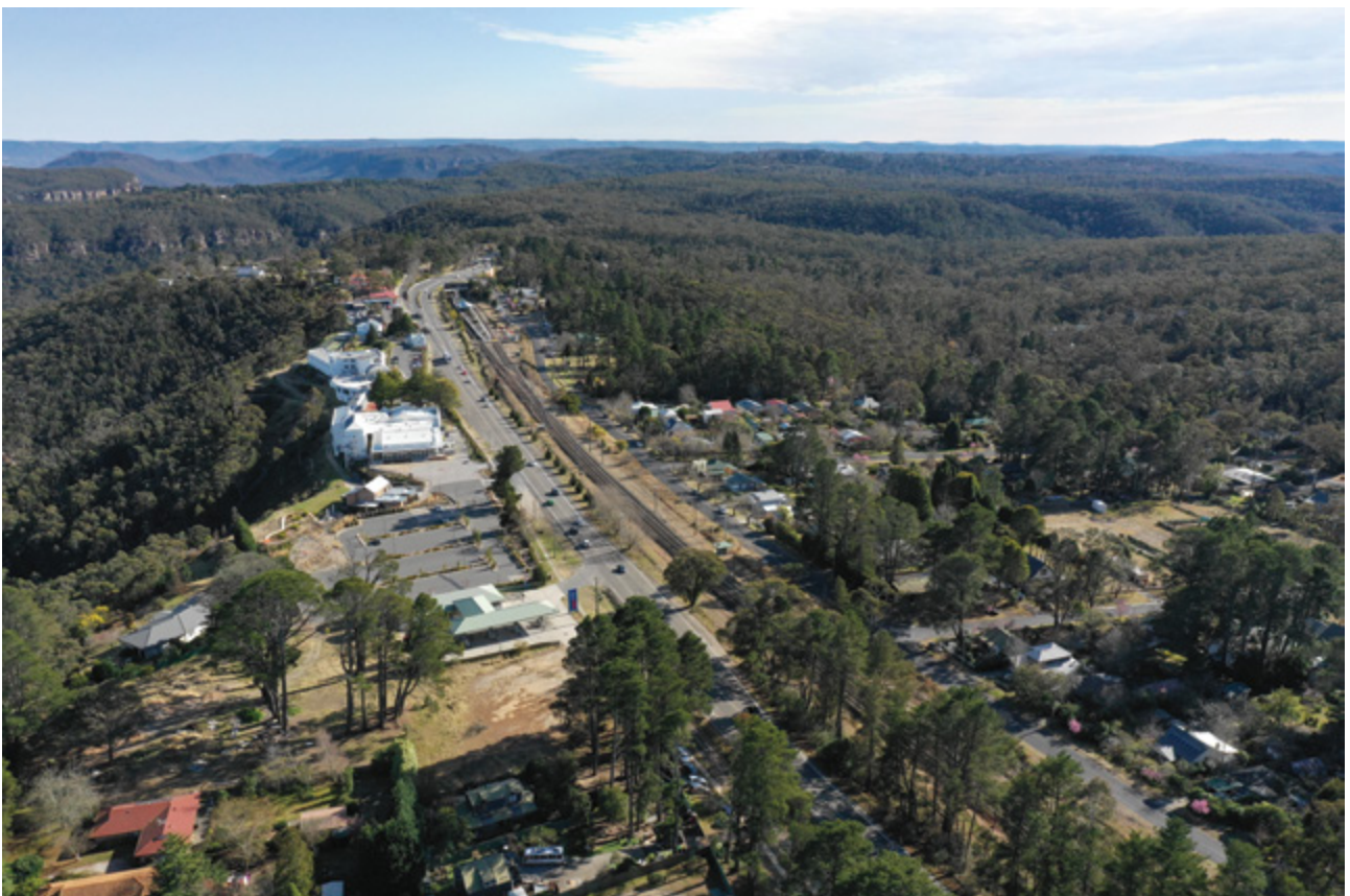
The Great Western Highway and rail corridor in Medlow Bath
