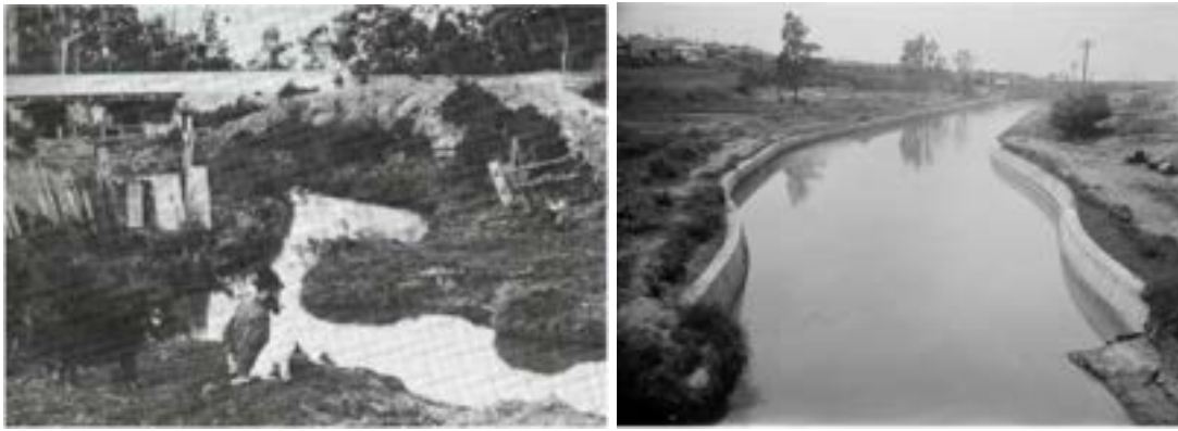
Figure 9: Left: Original condition of Iron Cove Creek near the Church Street bridge in 1890. Right: Section of Iron Cove Creek near Ramsay Street in 1929 after it had been canalised 23
