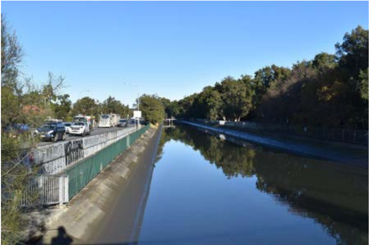
Figure 17: Southwestern view of Iron Cove Creek, the wide stormwater channel, from Timbrell Drive (Source: Artefact, 2023)
