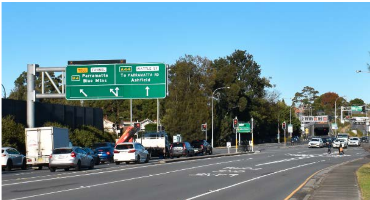
Figure 14: Southwestern view of Wattle Street intersection. The pedestrian bridge is proposed to replace the current street level pedestrian crossing (Source: Artefact, 2023)
