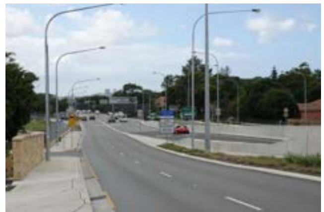
Figure 29 View east along Wattle St. with concrete walls of tunnel portal on the right, pedestrian path on the left & North Sydney commercial centre on the skyline
