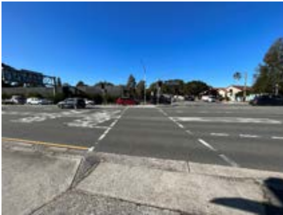
Figure 2-2 Existing Dobroyd Parade and Waratah Street signalised pedestrian crossing
