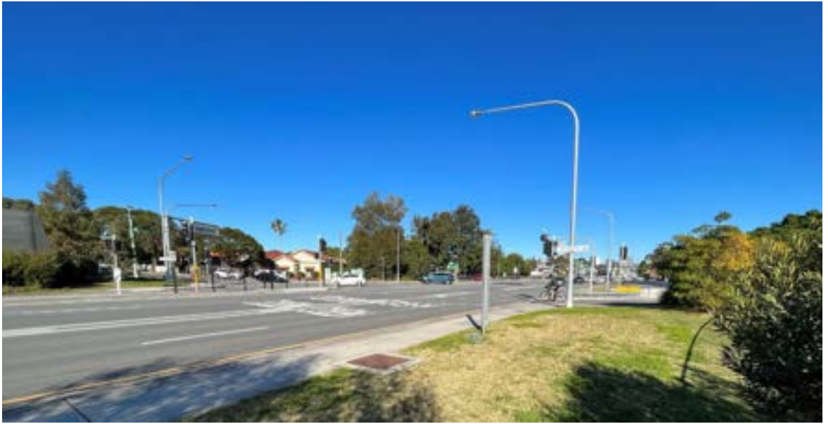
Figure 2-1 Existing Dobroyd Parade and Waratah Street signalised intersection
