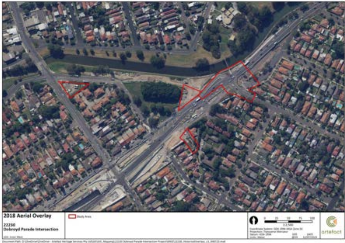
Figure 13: 2018 aerial photograph of the proposal area, showing construction for the WestConnex Project to the southwest
