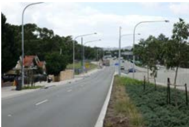
Figure 28 View east along Wattle St. with M4 exit on the right & Reg Coady Reserve on left
