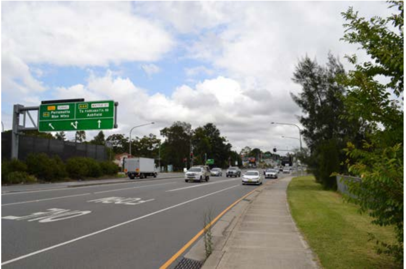
Figure 46 View along City West Link towards the WestConnex Portal Tunnel
