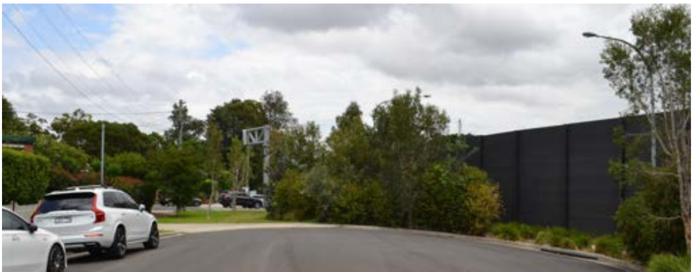
Figure 45 View from Dobroyd Parade looking west towards Waratah Street and towards proposed location of pedestrian bridge
