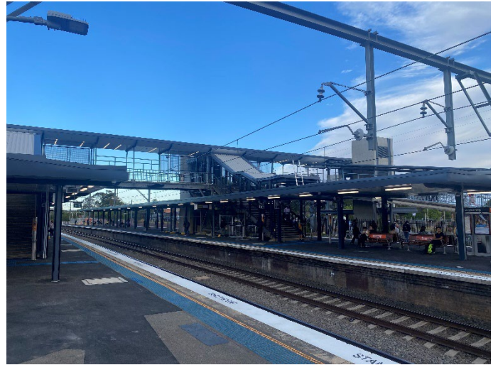
View of footbridge from Platforms 3 and 4
