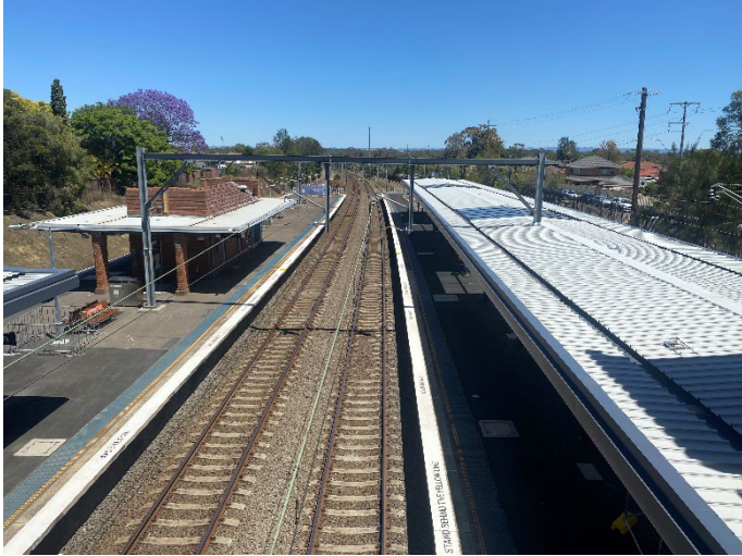
View of Platform 1 and 2 canopy from footbridge
