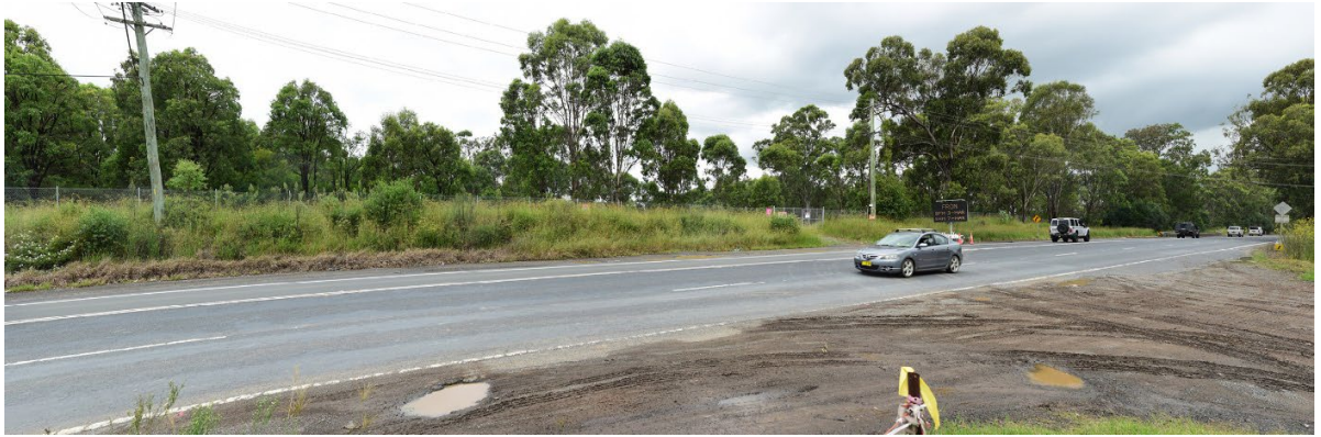
Figure 6-28 Existing view from Viewpoint 9 looking west along Elizabeth Drive (indicative only, subject to detailed design)
