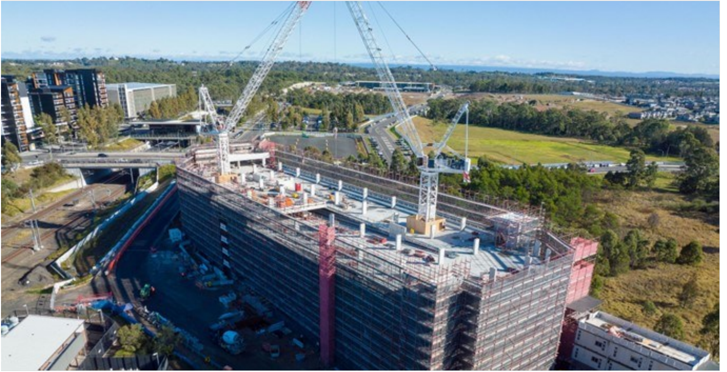
Progress photo of the commuter car park
