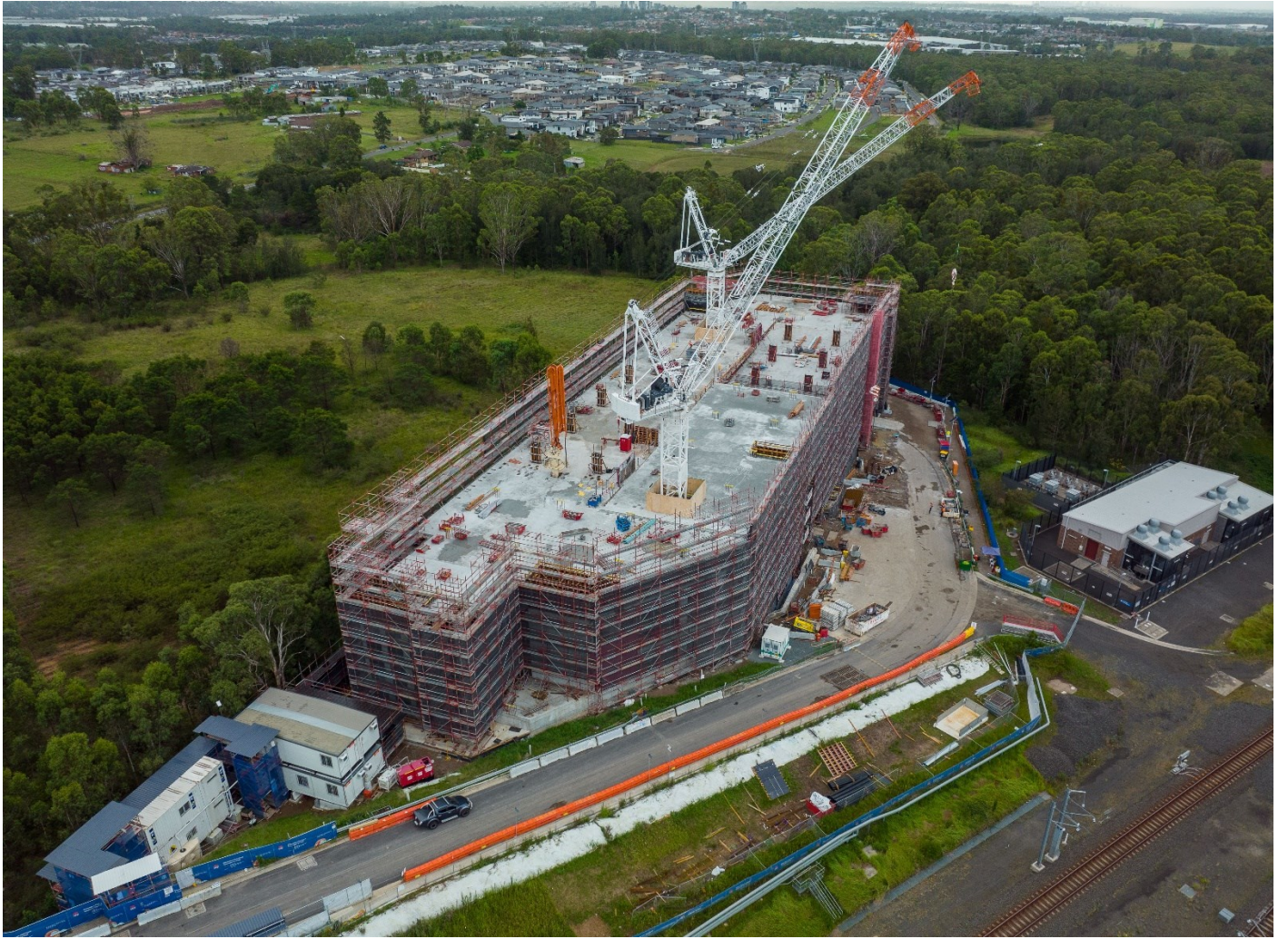
Construction progress on the Edmondson Park North Commuter Car Park
