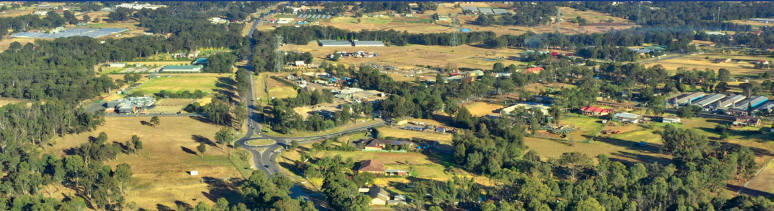
Elizabeth Drive (at Mamre Road intersection looking west)
