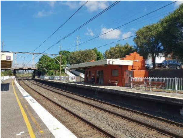
Photo 25 South-west-facing view of the western platform building
