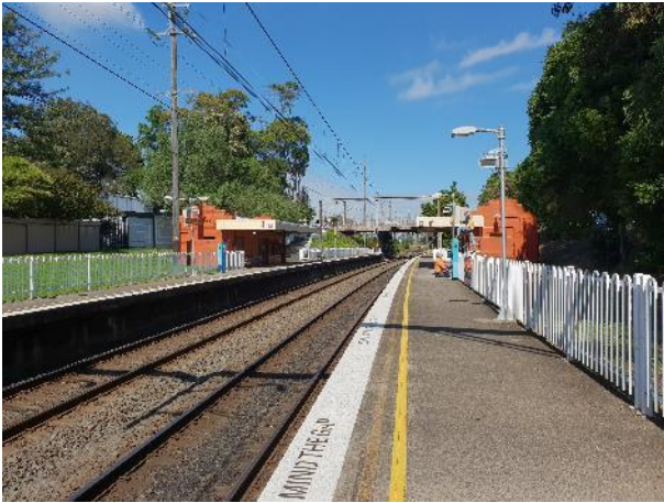
Photo 22 South-west-facing view of the two platforms and platform buildings
