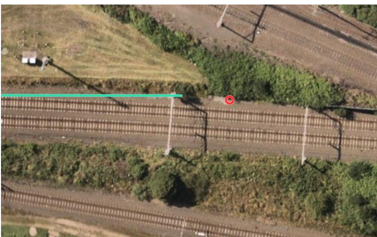
Photo 31 Guy anchor footing country side of the worksite (Source: Marsupial Lion, provided 28 June 2022)
