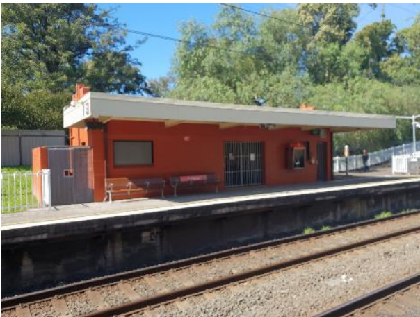
Photo 26 East-facing view of the eastern platform building
