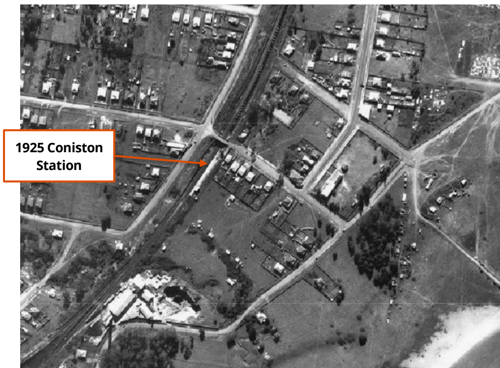
Photo 8 1938 aerial photograph of Coniston Station and surrounding suburban development (Source: (Wollongong City Council 2017a)
