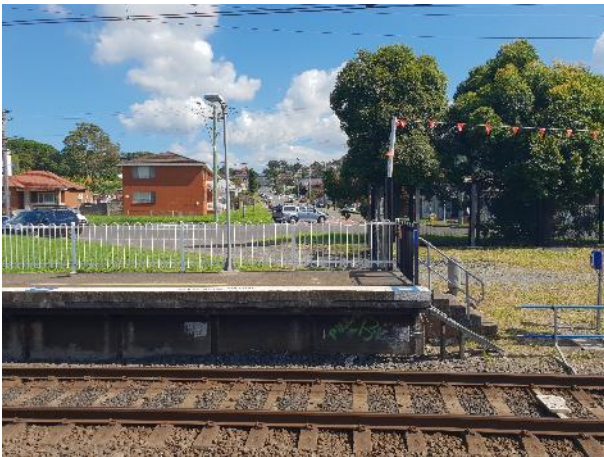
Photo 23 West-facing view of the western platform, northern end
