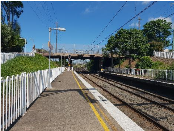
Photo 21 South-west-facing view of Coniston Station
