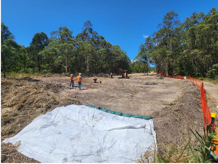
Image 1: Hollywood Heritage Salvage works
