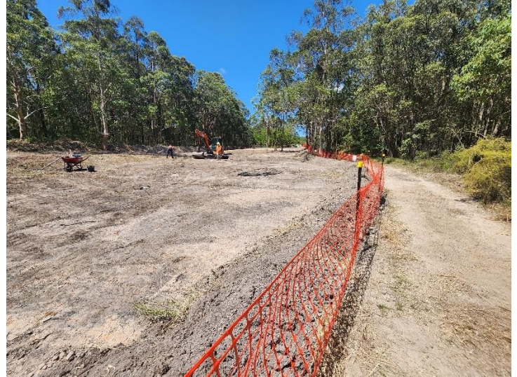
Image 2: Hollywood Heritage Salvage works
