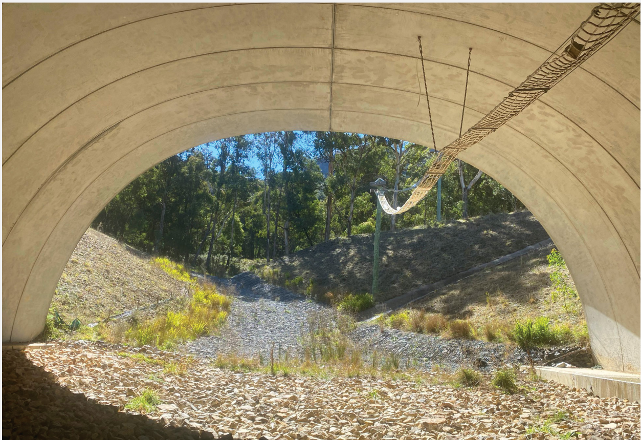
Existing combined drainage culvert and fauna underpass at Whites Creek
