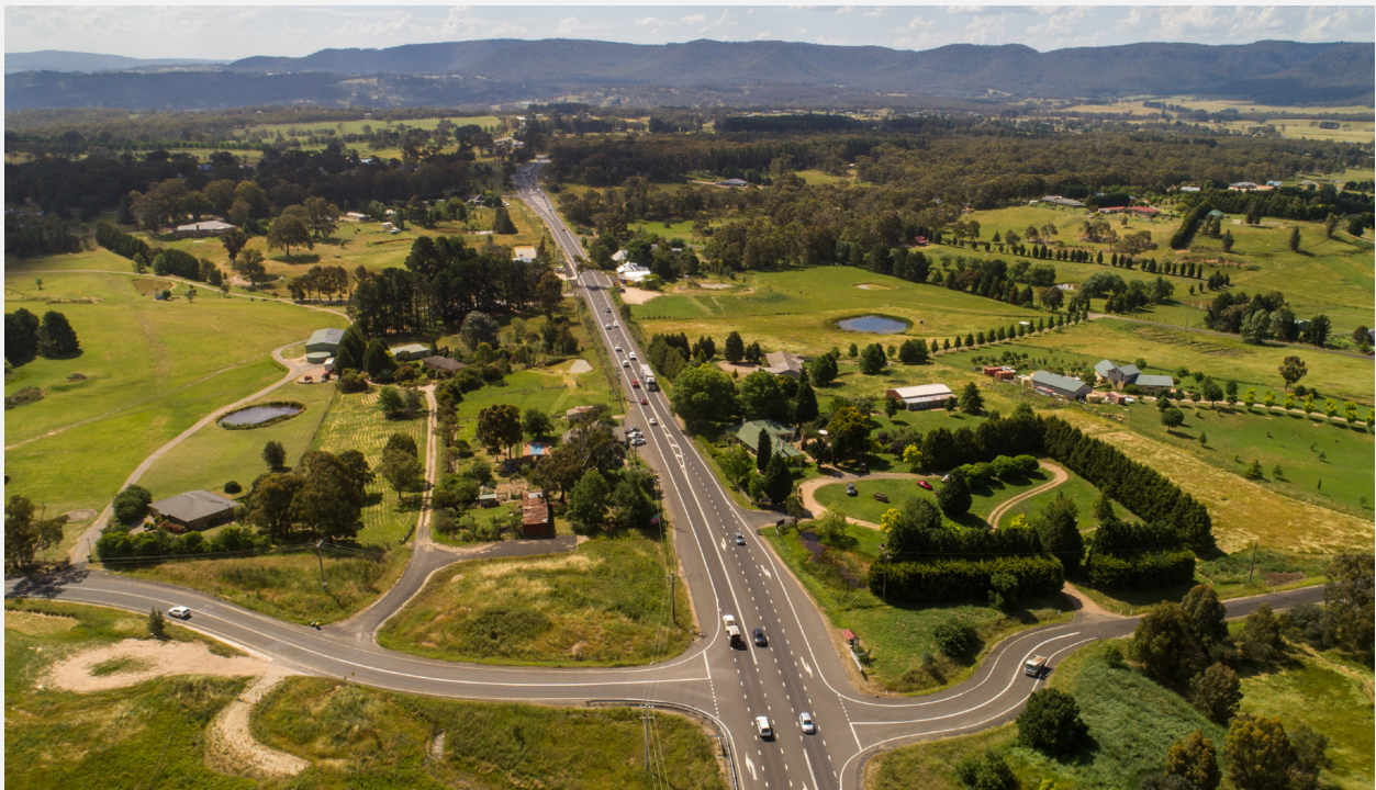
Great Western Highway looking west at Coxs River Road
