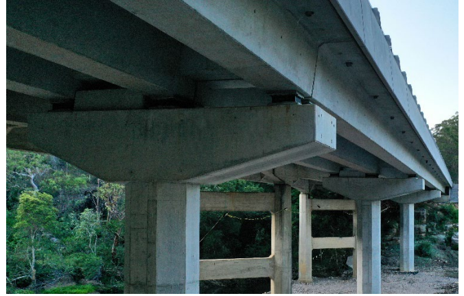
View under the new bridge
