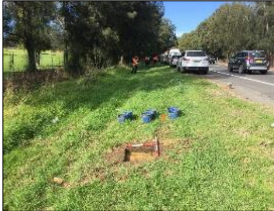
Plate 24. HLD PAD 6 facing south with TS 43 in foreground on road embankment with drainage ditch left.
