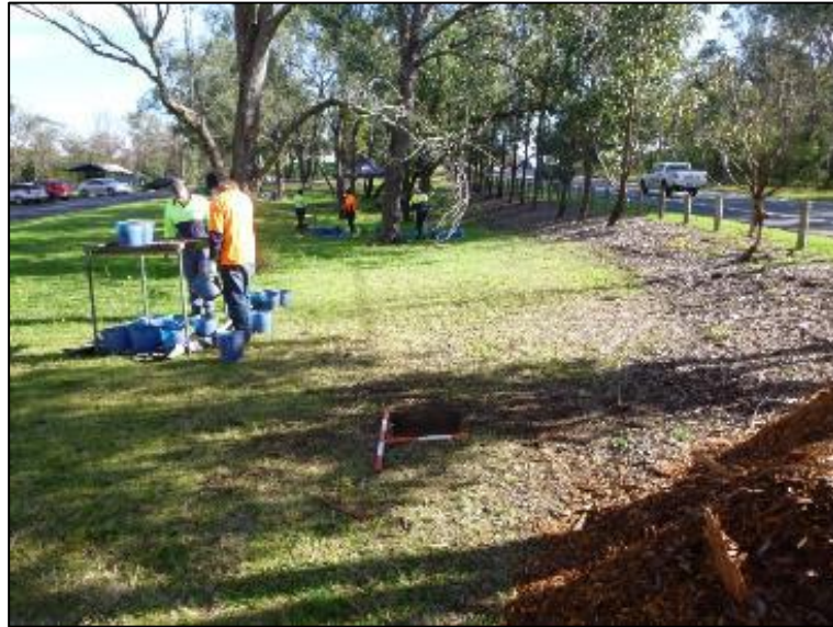
Plate 2. Excavation at HLD Site 1 (AS + PAD) showing TS 3 facing north.
