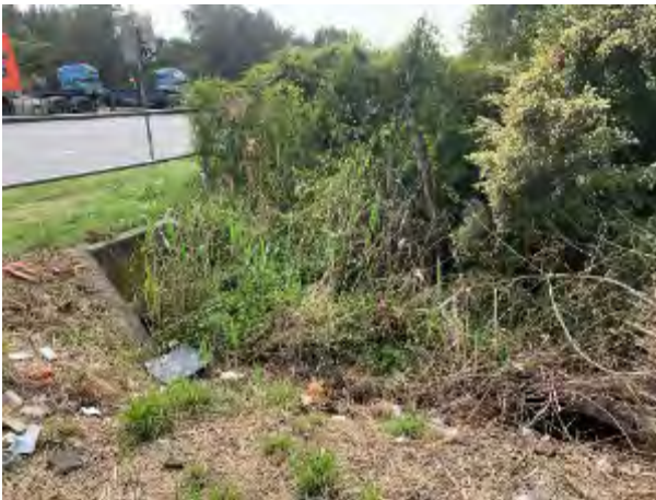
Photo 3.49 Aquatic Site 9 - A stormwater drain on the southern side of Milperra Road showing the pipe exit
