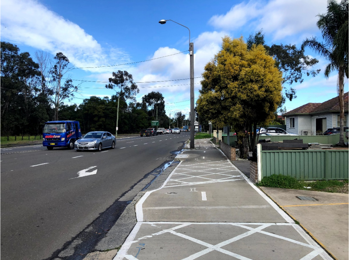
Figure 6-2 Residential properties on Henry Lawson Drive, south of Newbridge Road (facing south)
