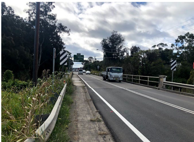
Figure 6-19 Henry Lawson Drive, north of the Auld Avenue Bridge (looking north)
