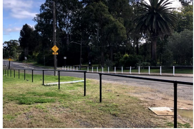
Figure 6-22 Auld Avenue (looking west)
