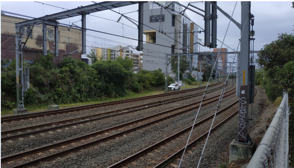
Figure 1.4 View from the eastern extent of the Proposal Area looking east. The Up and Down tracks of the Illawarra Main are the two tracks in the foreground.
