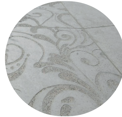
FIGURE 20 INTEGRATION OF ARTWORK ON CONCRETE APPROACH JETTY THROUGH SANDBLASTING
