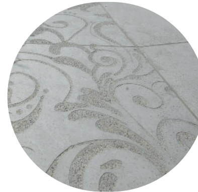
FIGURE 26 INTEGRATION OF ARTWORK ON CONCRETE APPROACH JETTY THROUGH SANDBLASTING
