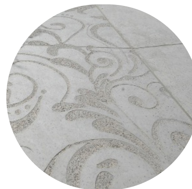
FIGURE 26 INTEGRATION OF ARTWORK ON CONCRETE APPROACH JETTY THROUGH SANDBLASTING
