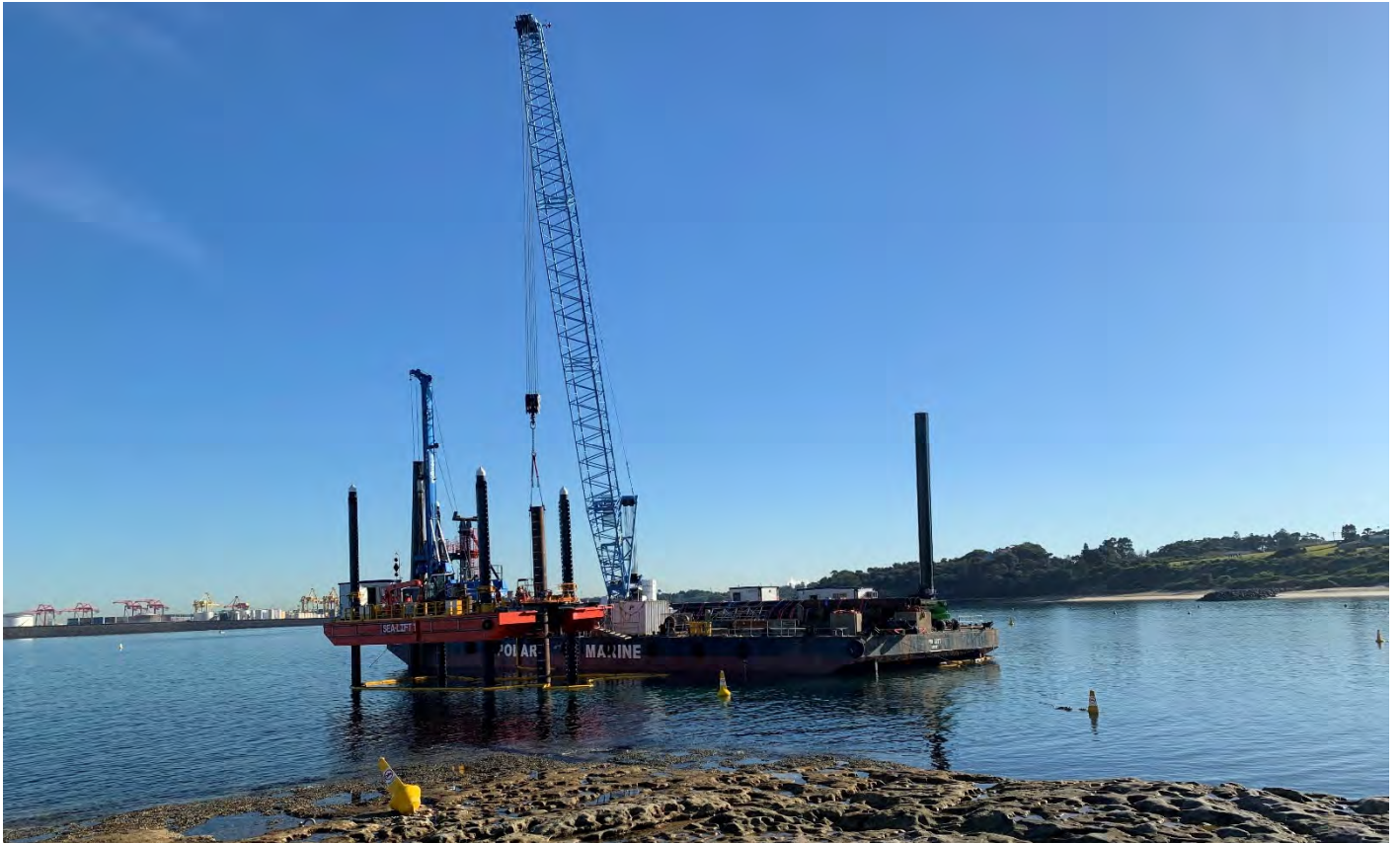
Image of barges and crane installing a pile at La Perouse.
