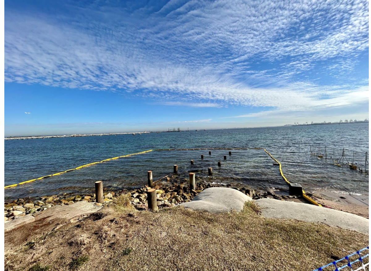
Silt curtains used to contain sediment if produced
