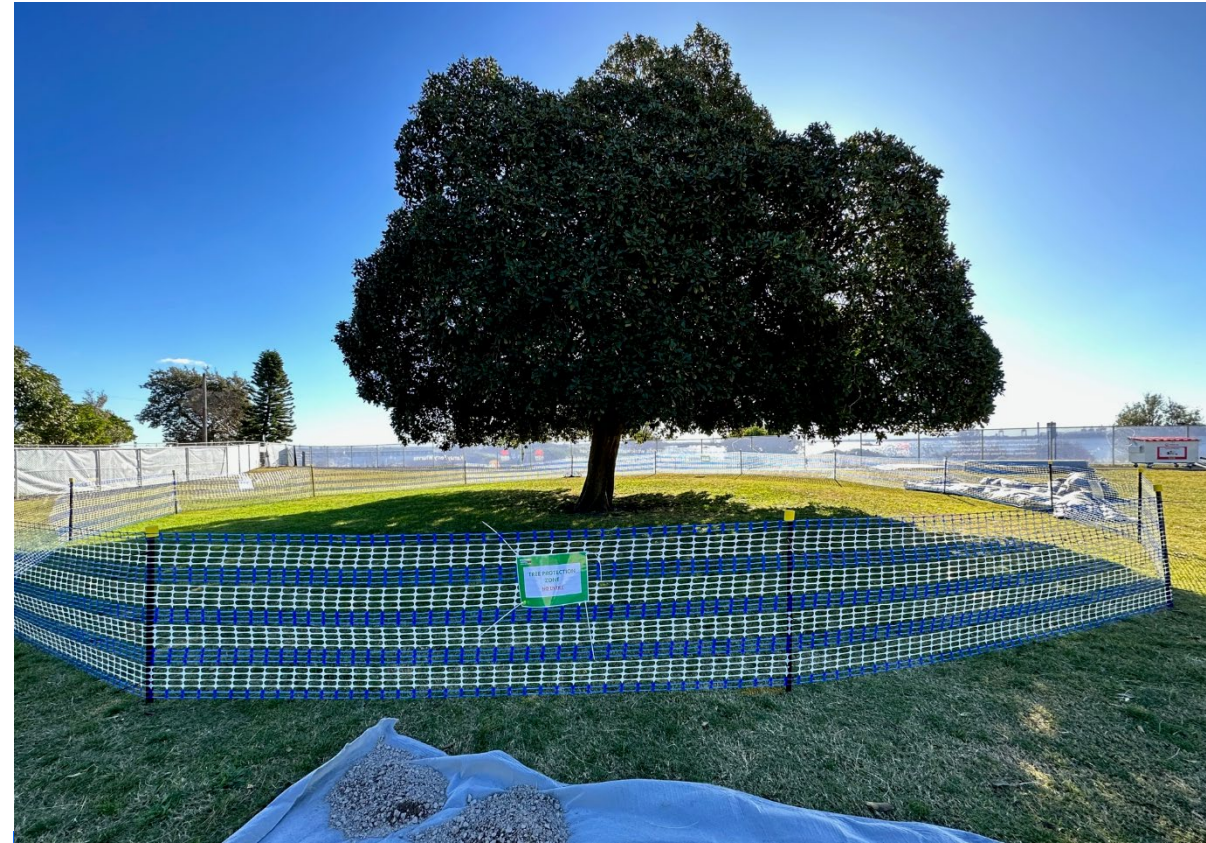
Tree protection installed
