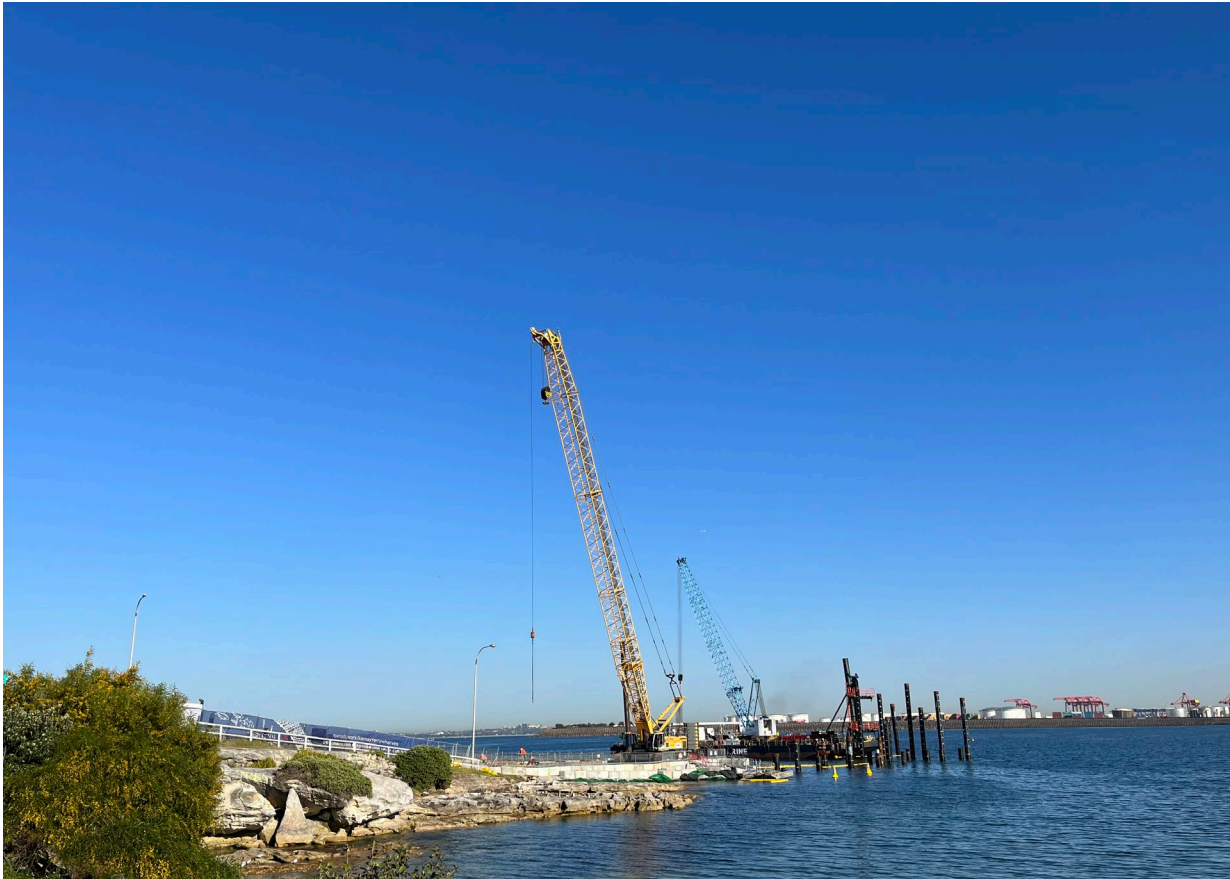
View of the piling equipment at La Perouse
