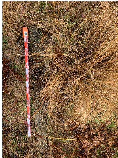
Plate 20: Secondary example of concrete edging in Subject Area
