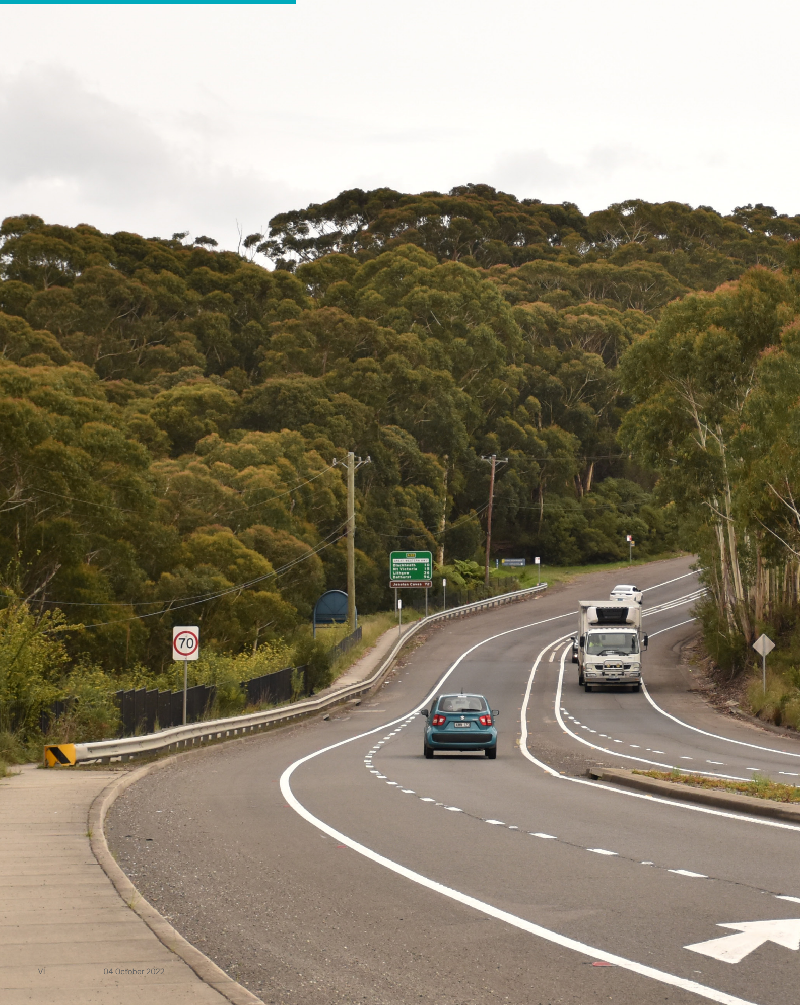
Existing view of the Great Western Highway looking north from Rowan Lane
