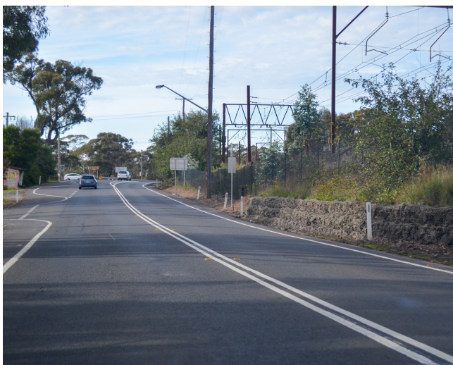
Figure 3-1 View along the Great Western Highway looking south toward the rail corridor upon exit of Blackheath
