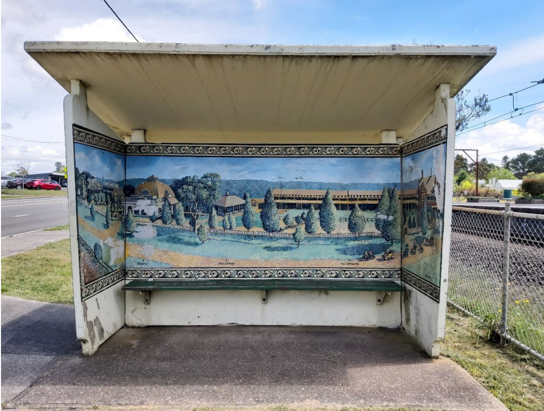
Figure 6-17: Bus shelter looking north, showing interior mural (RPS, 2021b)
