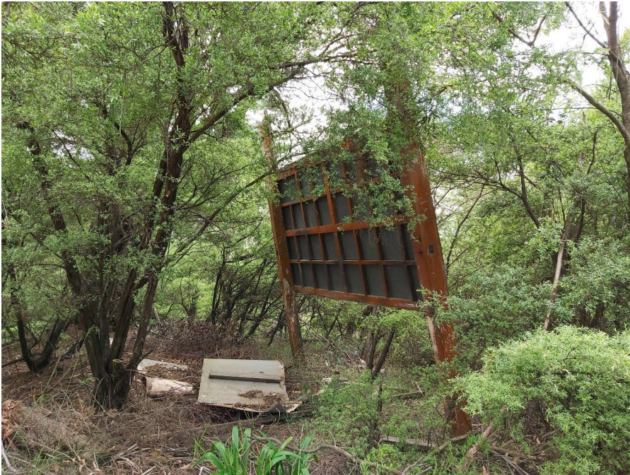
Figure 6-19: Rear of advertising sign, looking east (RPS, 2021b)
