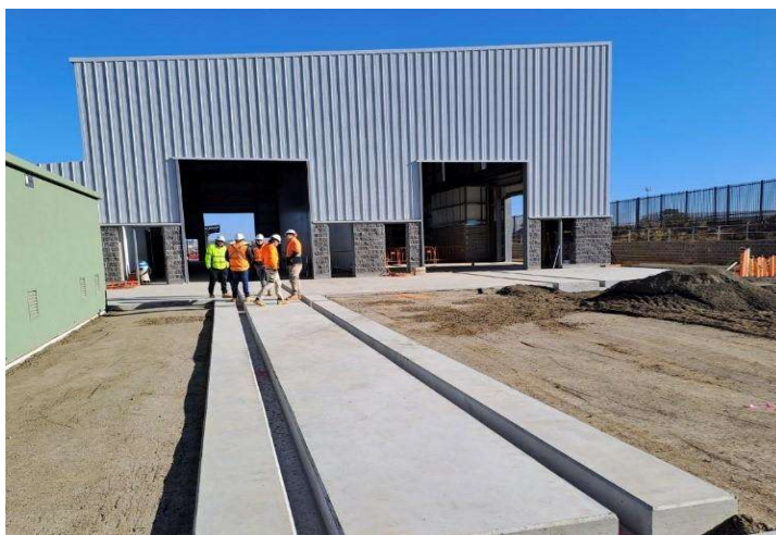
Embedded rail system ready for the rail installation.
