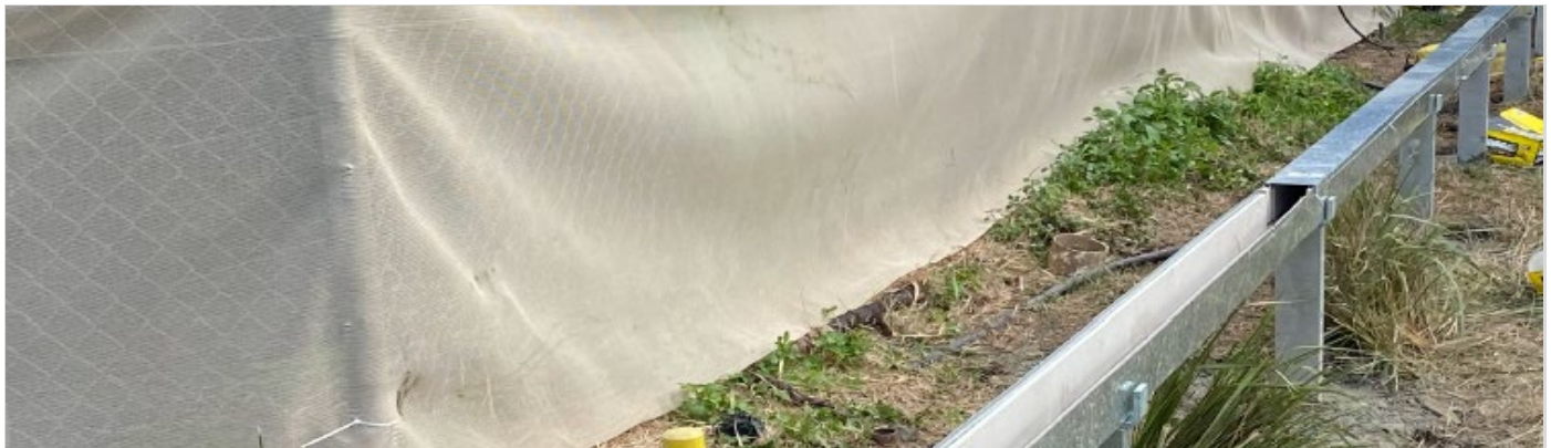
Galvanised steel trough installed on Burren Street near Macdonaldtown Stabling Yard in May. In July we will feed cables through the trough to support new signalling infrastructure inside the rail corridor.
