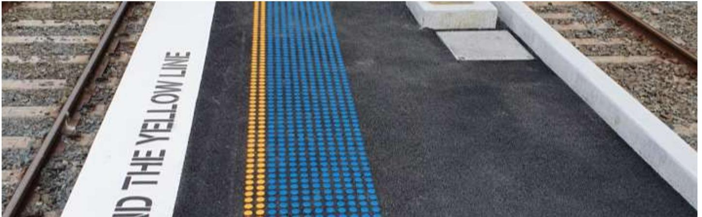
Section of platform extension including new asphalt, paint and tactiles at Kiama Station – August 2021
