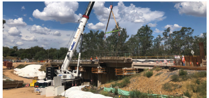
Road segments lifted from northern side of Mandagery Creek Bridge
