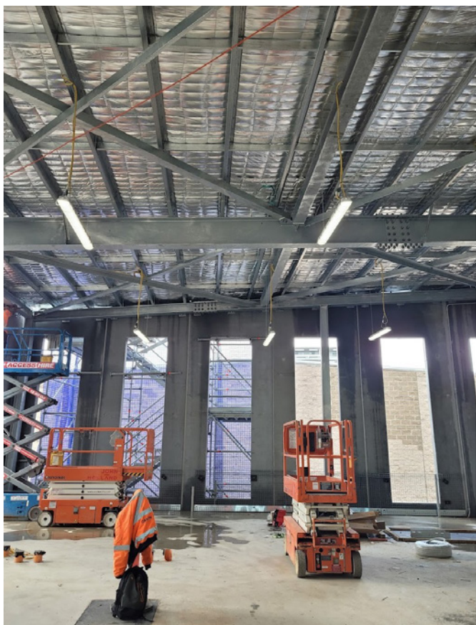
Electrical fit out of the interior of the substation has commenced
