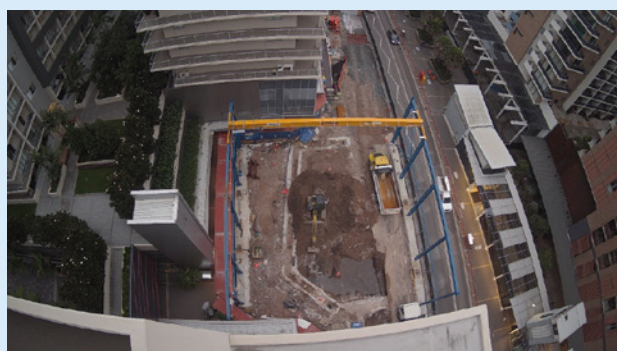
Progress at Mascot Station
