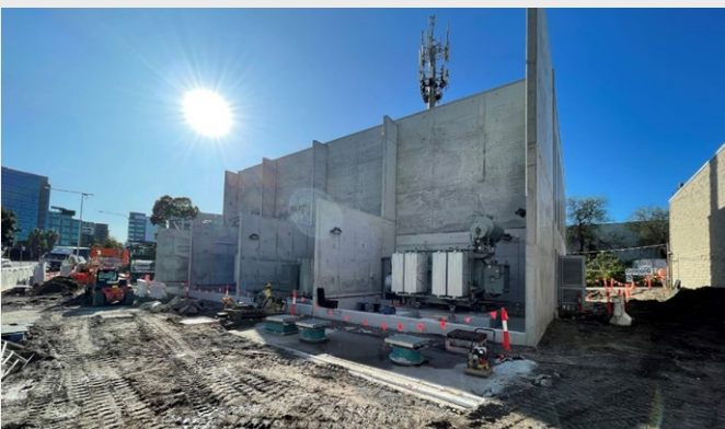
The substation at 166 O'Riordan Street taking shape.
