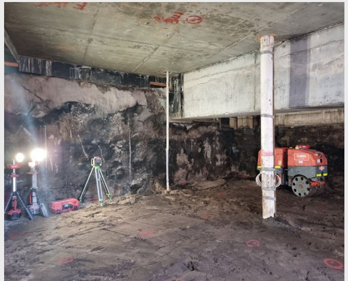
Excavation of the new western station entry.
