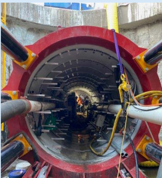
A view into the cable tunnel from the future substation site.
