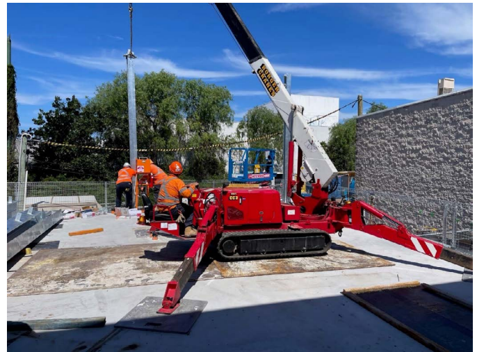
Steel fixing at the future substation building at 166 O'Riordan Street, Mascot.
