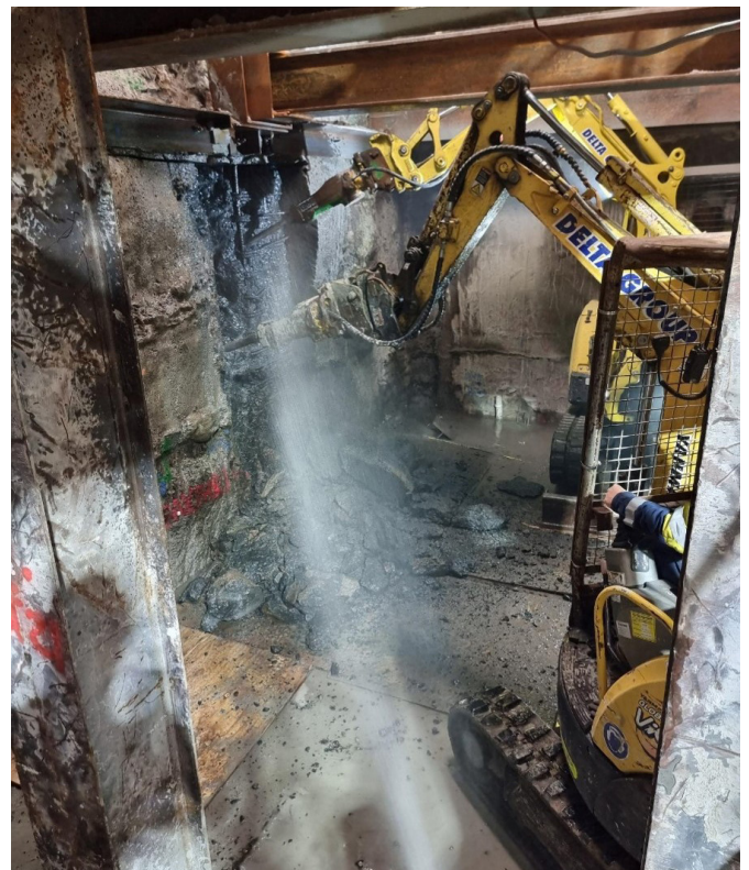
Excavator breaking through diaphragm wall.
