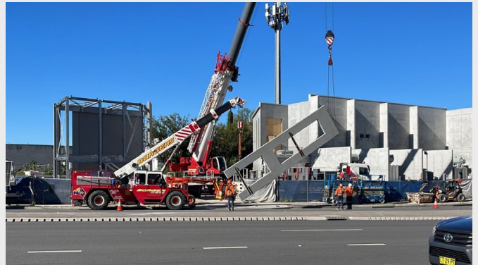
Precast panels being craned into the 166 O'Riordan Street substation site.
