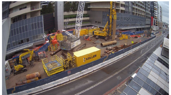
Work progressing on construction of the new western station entry.
