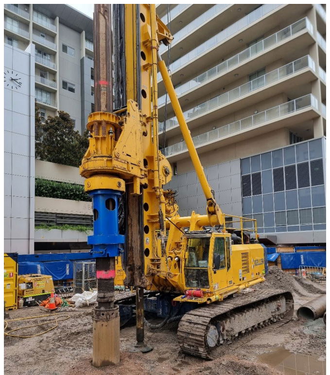
Piling works were completed in February.
