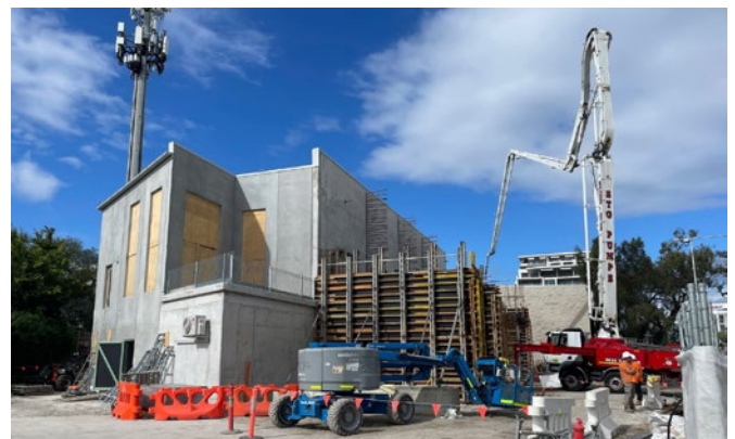
Progress on the substation at 166 O’Riordan Street
