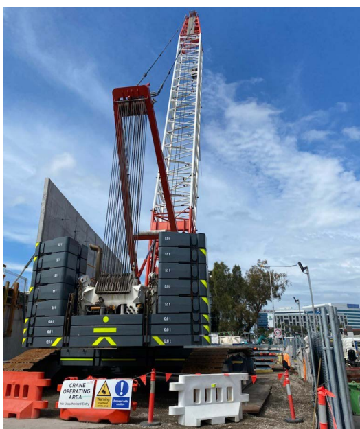
The large 280 tonne crane currently working at the future substation site.
