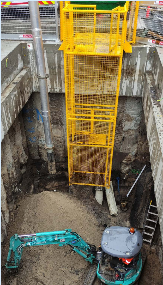
Looking into our tunnelling retrieval shaft on Bourke Road.
