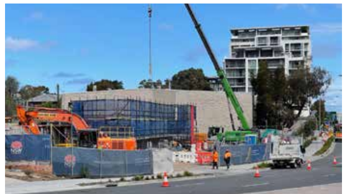
Work continues on the substation at 166 O’Riordan Street
