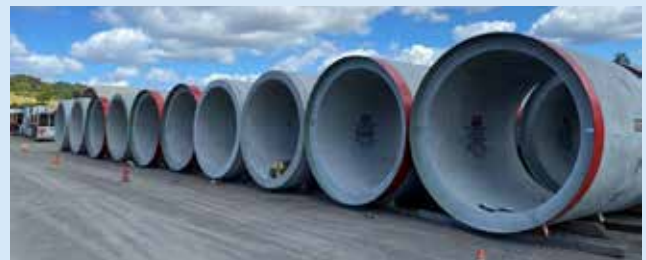
Pipe sections which will form substation Cable tunnel, arrived safely at Port Kembla last month
