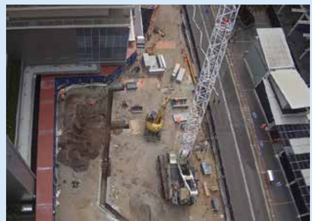
The crane in position preparing for the retaining wall work
