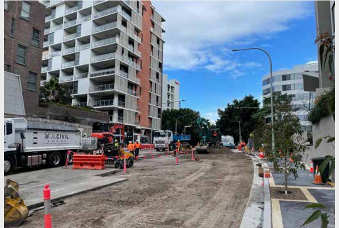
Work in progress: pathway complete and preparation works for asphaltting.
