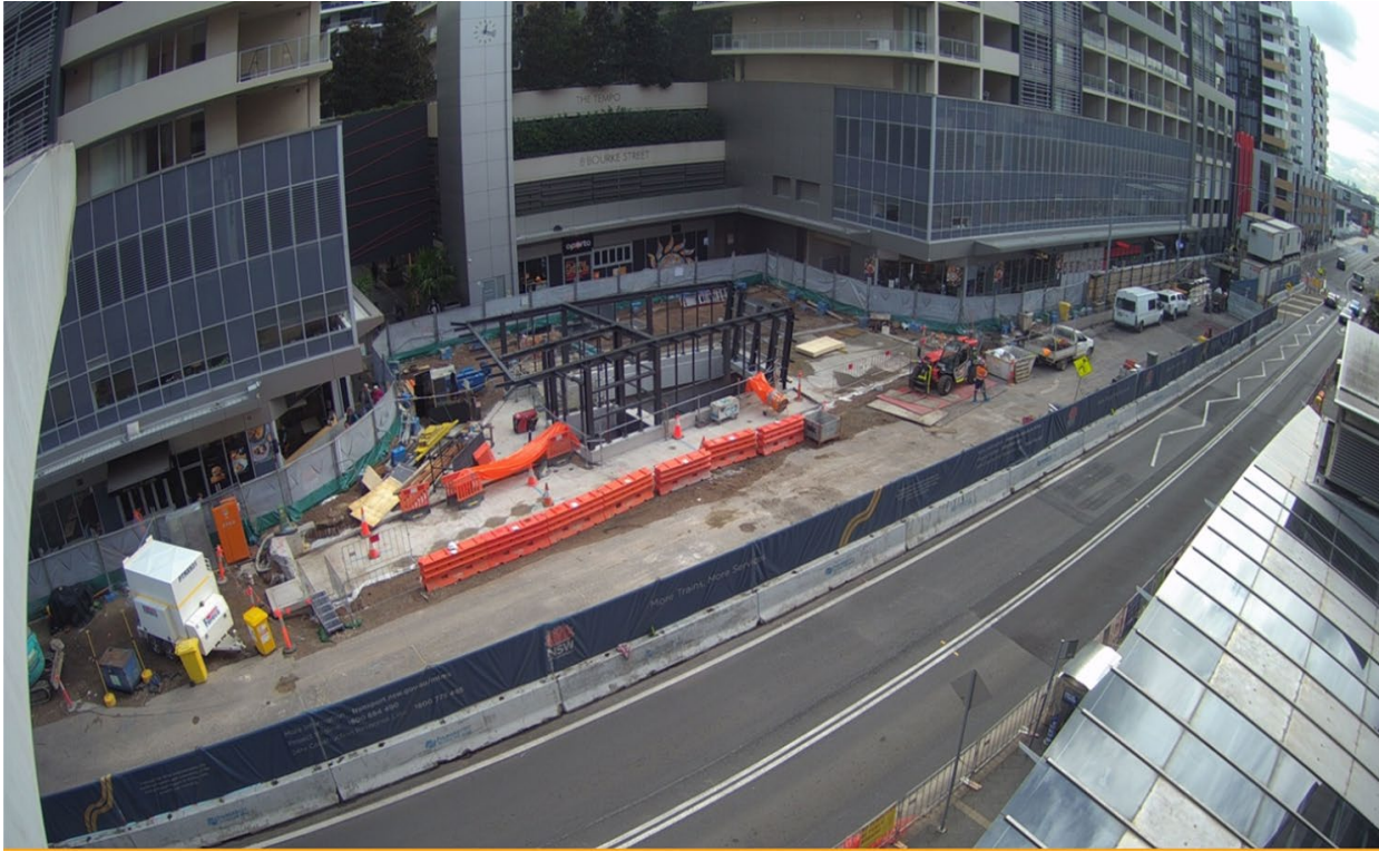
Structural steel work for the new western entrance
