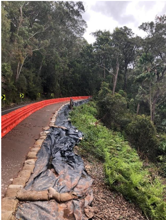
Figure 3-1 Road slumping on McKell Avenue
