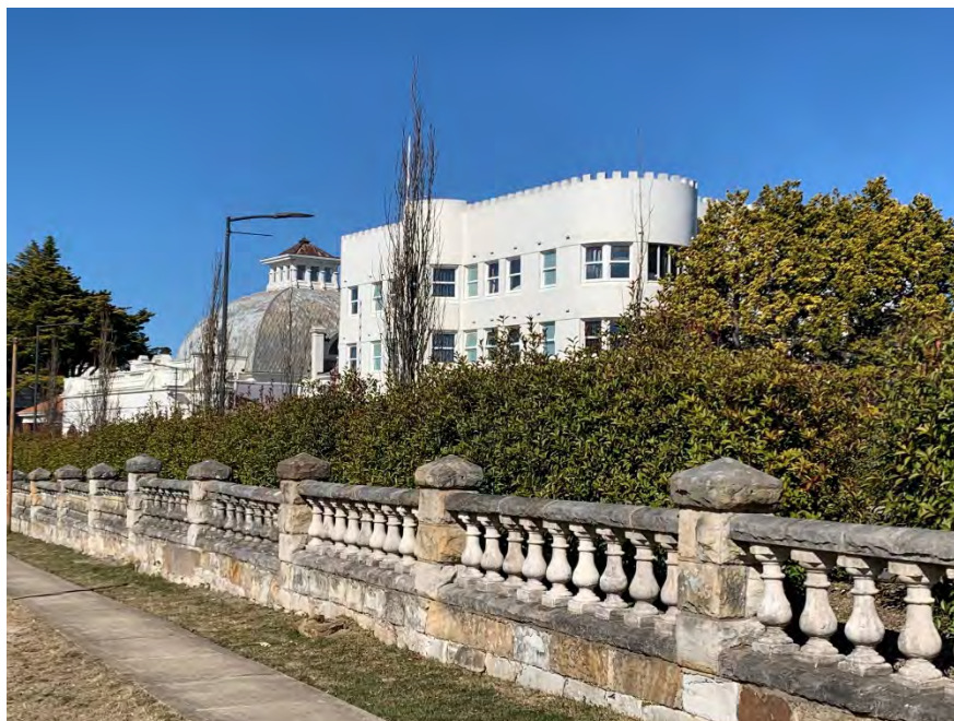
Figure 10: sandstone wall of the Hydro Majestic, containing physical impact but not visual impact
