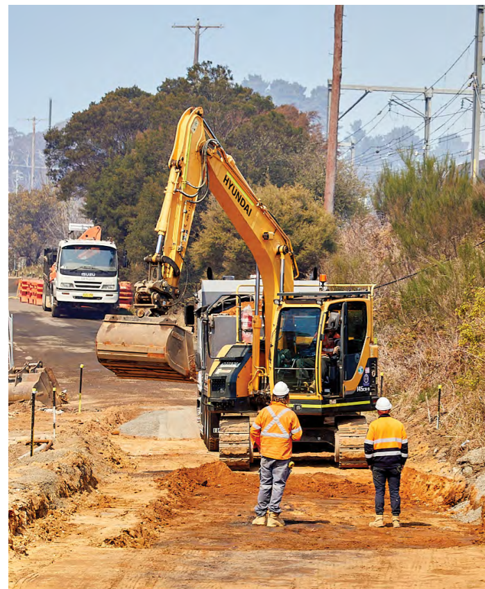
Railway Parade road foundation preparation
