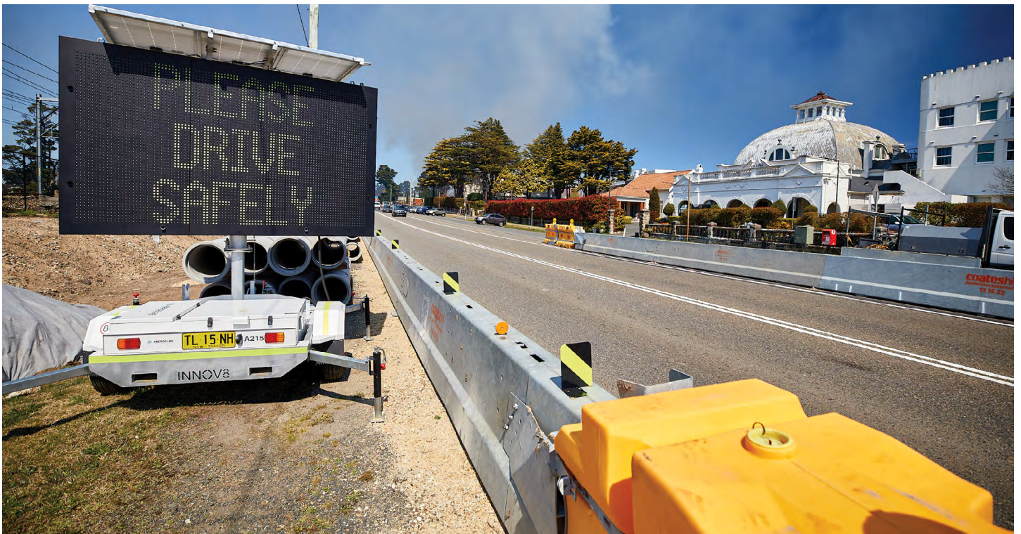
Barriers in place on the highway
