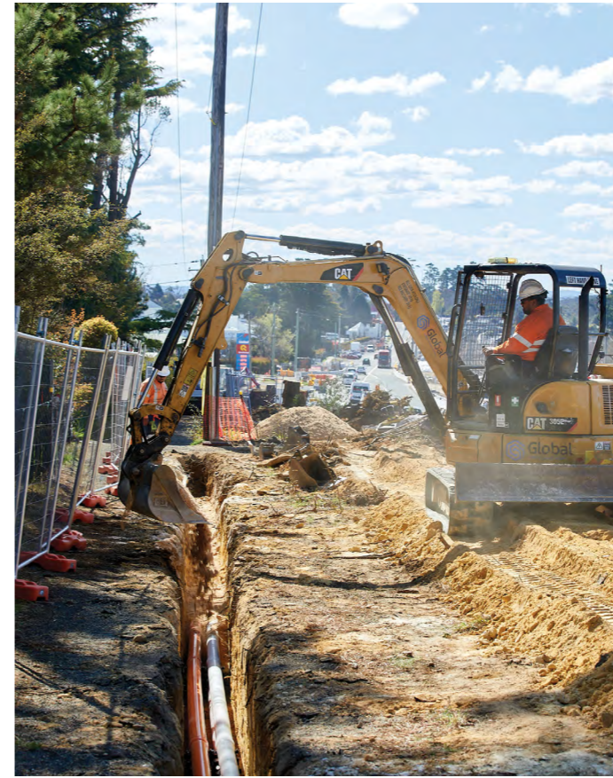
Excavation underway to relocate utilities along the Great Western Highway
