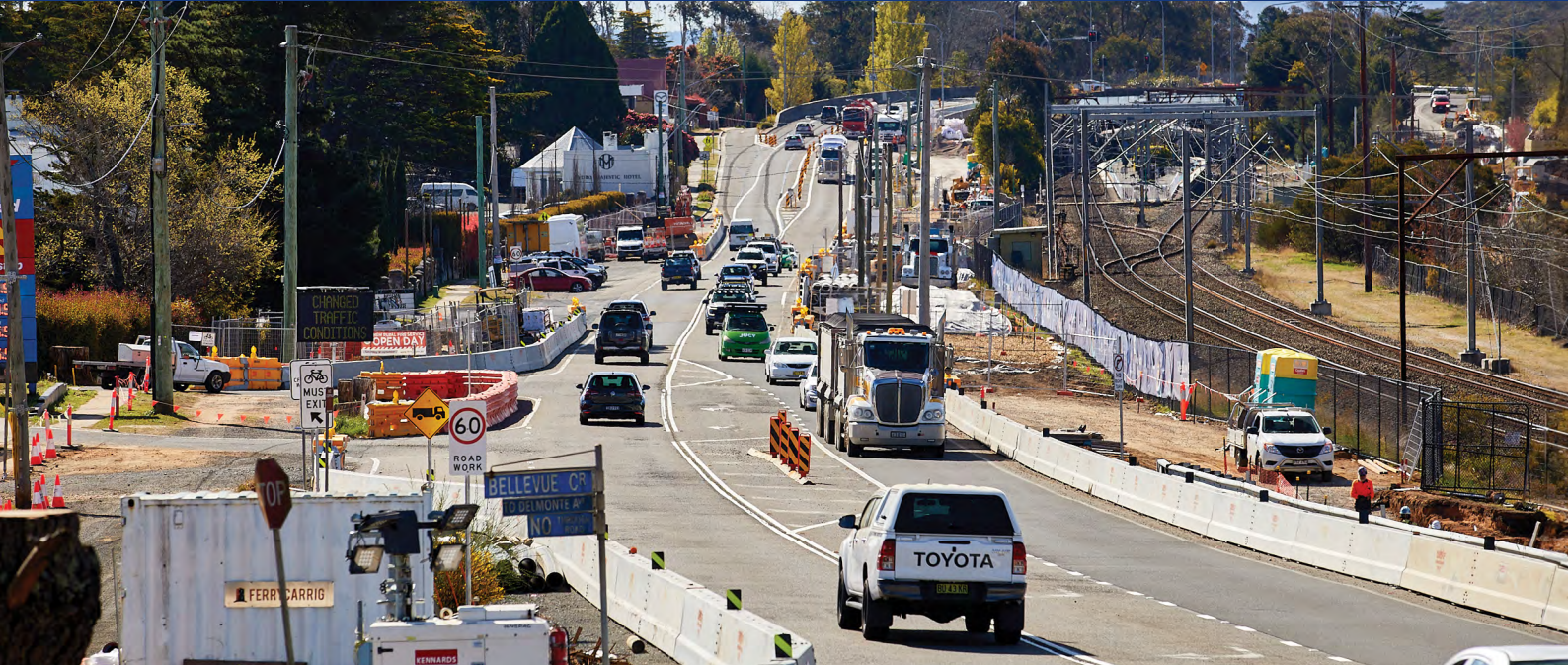
Roadwork underway on the Great Western Highway at Medlow Bath
