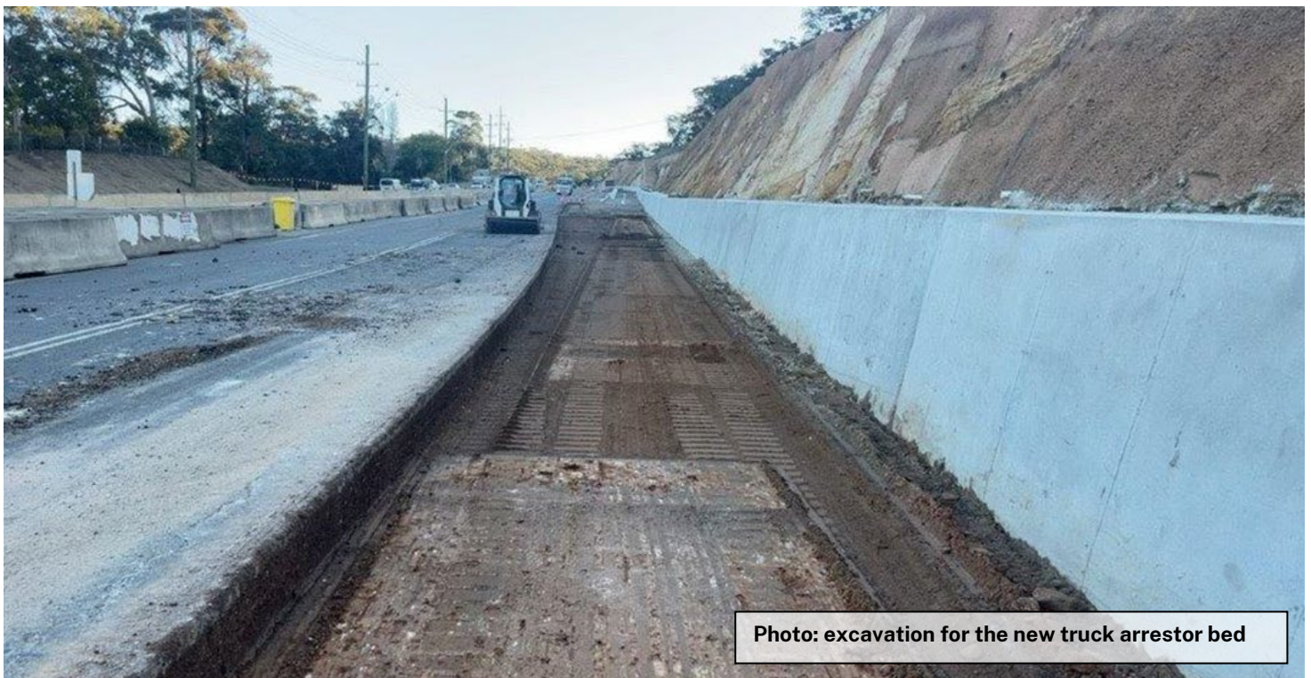
Photo: new concrete median dividing the new east and westbound lanes near Ingleside Road (looking west)
