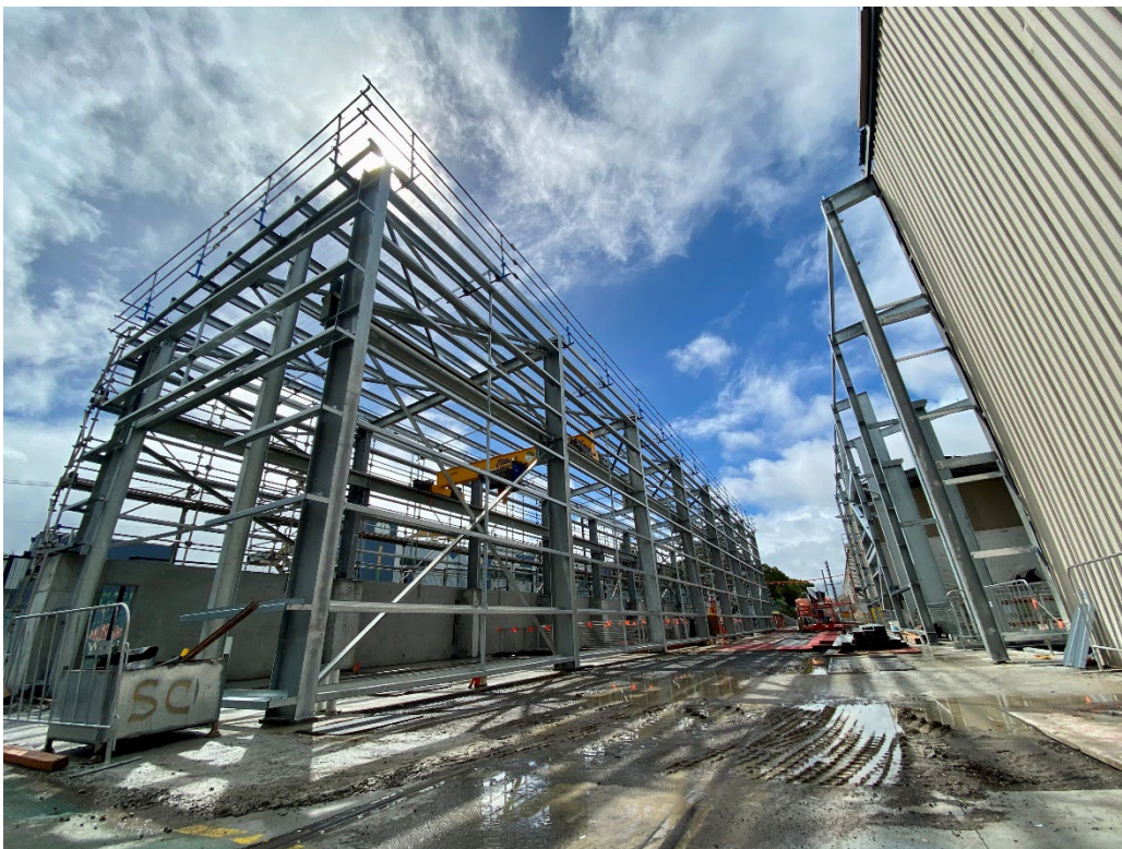
Steelwork progress for the Mortdale Maintenance Centre
