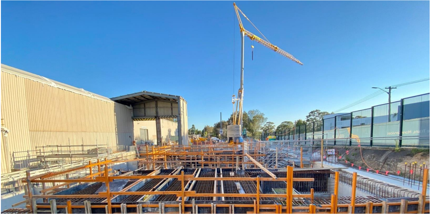
Construction of the Mortdale Maintenance Centre – November 2021
