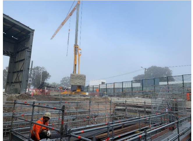
Image showing progress inside the Mortdale Maintenance Centre, taken in June 2021.
