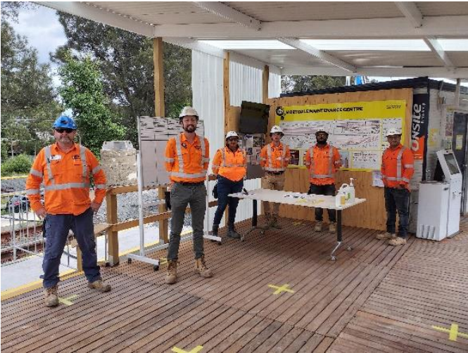
The Mortdale Maintenance Centre project team and subcontracted concrete supplier meet on-site to identify a more sustainable approach to construction.
