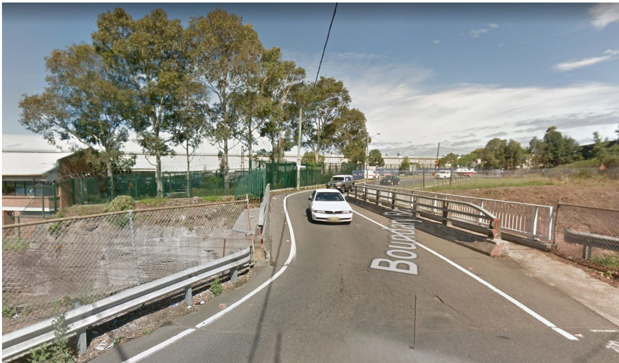
Figure 6.1 Boundary Road bridge facing south east towards Mortdale Maintenance Centre (Source: Google maps)
