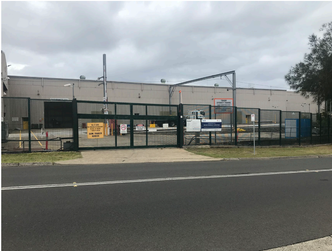
Figure 1.4 View of the Mortdale Maintenance Centre from Hurstville Road looking east. This photograph shows the existing entry/exit gate which would become entry only. A new exit gate would be constructed to the right of the frame.
