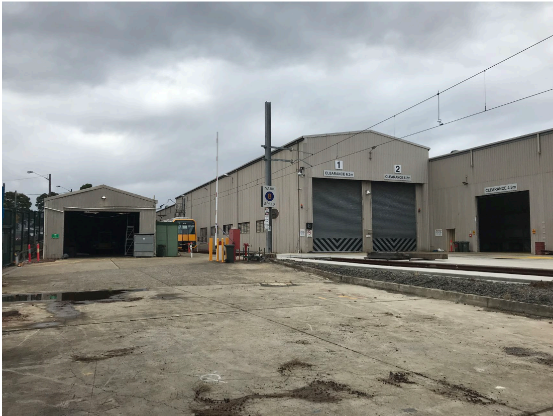
Figure 1.3 Photograph adjacent to the western boundary, facing north, showing the existing maintenance sheds. The shed on the left is to be demolished and replaced with a new bogie exchange shed, similar in style to the shed on the right.
