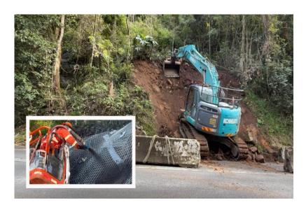
A long-reach excavator was used to remove loose material and drill the soil nails, while workers accessed the steep slope from an elevated work platform (inset) to complete tasks like applying shotcrete.
