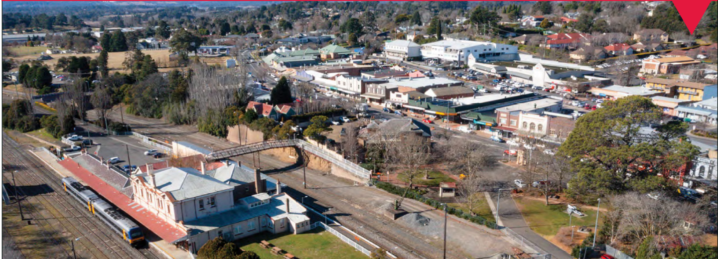
Moss Vale Station.
